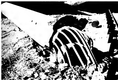
Photo 14. Failure at base of column supported on a single 6-foot-diameter cast-in-drilled-hole pile, Golden State Freeway and Foothill Freeway interchange [4].
